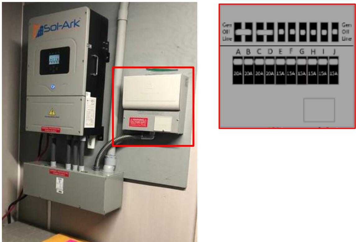
Figure 7.0 – Transfer Switch Kit
