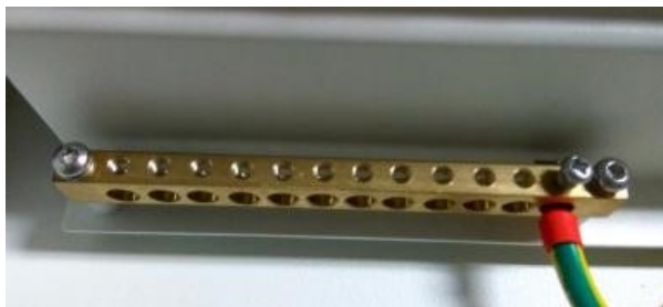
Figure 3.9 Grounding terminal block on the metal bracket
