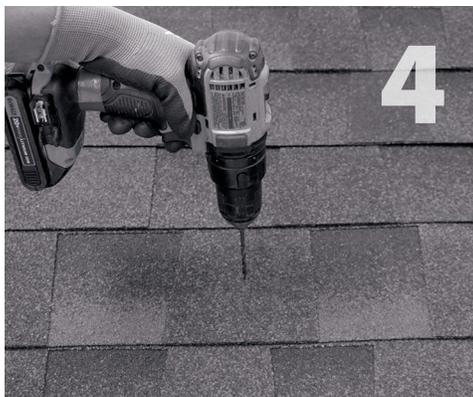
4 Drill pilot holes into roof and rafter using a with 7/32" bit, taking care to **drill square to the roof**. Do not use mount as a drill guide. Drill each hole 2.5" deep into rafter.
