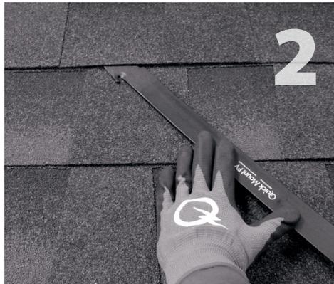
2 Carefully lift composition roof shingle with roofing bar, just above placement of mount. Remove nails as required and backfill holes with approved sealant. See "Proper Flashing Placement" on next page.
