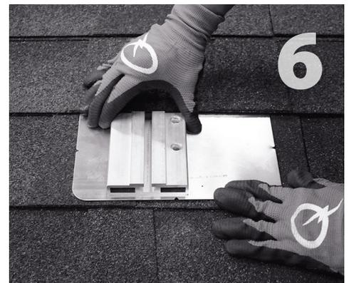
6 Slide flashing into position.
