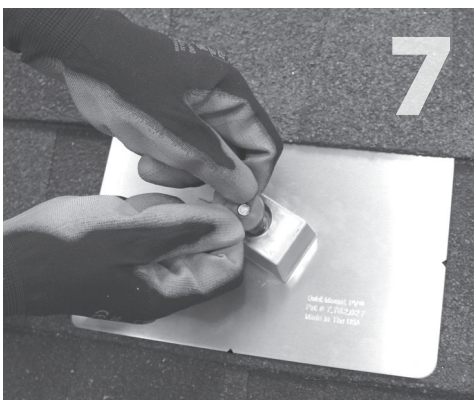
7 Insert EPDM rubber washer over hanger bolt into block.
