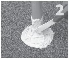
Chem Link's M-1. Coat the QBase, bolts base of both E-Curb sections. and post with M-1 to 3" above roof line.
