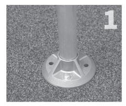
Install QBase to structural member. For more details refer to the QBase Low Slope installation instructions.
