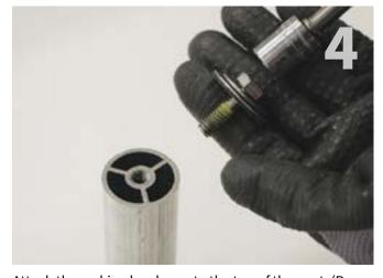
Attach the racking hardware to the top of the post. (Be sure to seal off the post from weather exposure with the sealing washer in the interim before racks are installed.) Flash the mount with a flashing appropriate to the roof type. (See previous page.)
