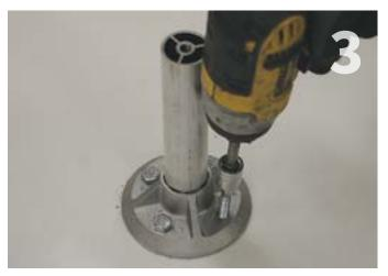
Prior to attaching the base to the roof, place the grade-8 hex bolt in the bottom of the base and screw the post in. This is easier than adding the post after securing the base to the roof. Attach the base/post assembly to the roof with selected fasteners.
