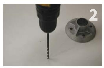
Drill pilot holes as required for selected fasteners. Make sure to hold the drill square to the roof. Fill the pilot holes with a sealant compatible with roofing materials.
