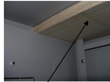
3/4" Piece of wood added as support
