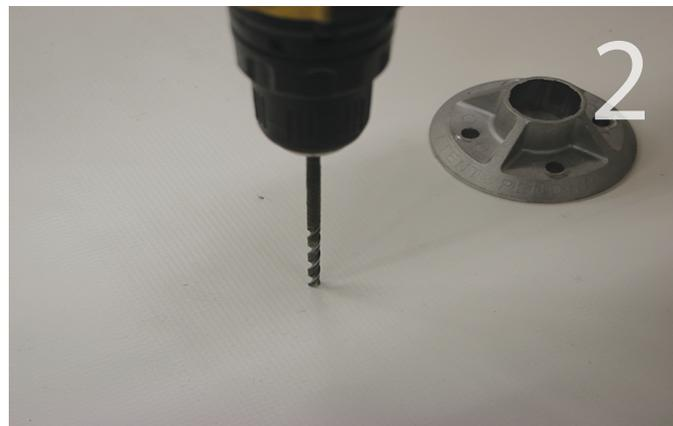
Drill pilot holes for the fasteners based on American Wood Council recommendations. Make sure to drill perpendicular to the roof. Backfill the pilot holes with a sealant compatible with roofing materials.
