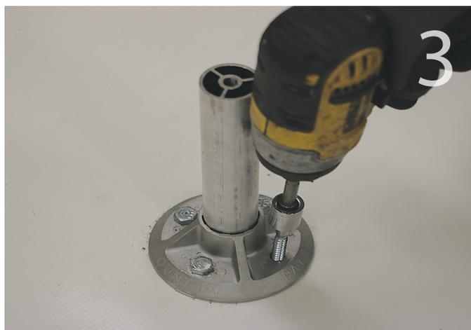
Prior to attaching the base to the roof, place the grade-8 hex bolt into the bottom of the base. Fully seat the post into the base, using slip-joint pliers if necessary. Attach the base and post assembly to the roof with the fasteners specified for the project.
