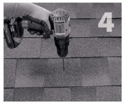
If attaching with lag bolt use a 1/4" bit (Lag). Use a 1/4" bit (ST) for attaching with the structural screw. Drill pilot hole into roof and raft er, taking care to drill square to the roof. Do not use mount as a drill guide. Drill a 2" deep hole into
