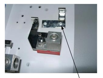
Remove two bolts holding small busbar. Remove small busbar from PV Positive lug **Step 2:** Remove PV Positive Combined Out and Negative box lugs
