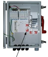
Install block. Refer to torque chart on page 4. Use screws removed in step 1
