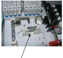
Install Negative out block with screws removed in step 1. Tighten onto busbars. Refer to torque chart on page 4. Step 5: Reinstall block
