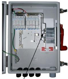
Install Supplied PV Positive busbar for 2 inverter configuration. Oriented as shown.
