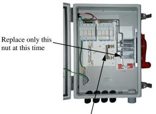
Remove Positive jumper busbar from switch, set aside, it is not used in this configuration. Replace nut on lowest position only
