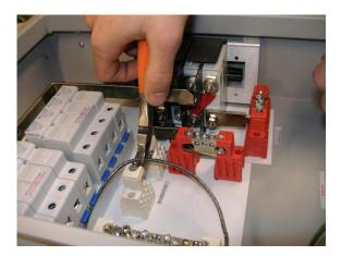
The wiring varies based on which configuration is used, so the wires will need to be cut to length. Refer to the wiring diagrams beginning on page 17 for details on your configuration
