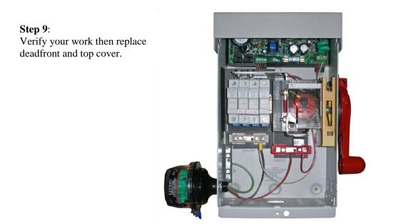
MNPVHV4 TYPE 3R Shown wired with MNDiscoPSB power supply board and MNSPD surge protector.
