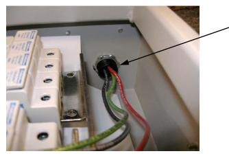
Remove the hole plug from the side of the combiner. Remove the nut from the MNSPD. Pull the wires through the side of the combiner and secure with the supplied nut. Insure that the silicone washer is installed on the outside of the chassis to maintain watertightness.
