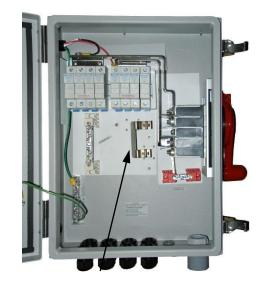
Remove Positive jumper busbar from switch, set aside, it is not used in this configuration. Replace nut on lowest position only.
