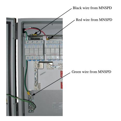
Connections for Non-Isolated. Refer to the wiring diagrams starting on page 17 for more information or If adding a second MNSPD600 (not included).
