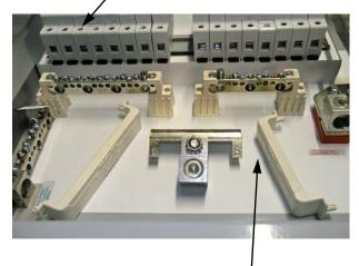
Remove terminal block covers by lifting gently
