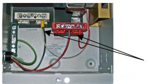
**Step 7a**: Strip the other end of the red and white wire about  $\frac{1}{4}$ ". Install the red wire into the red terminal block. Put the white wire along with the black wire from the MNSPD into the ferrule and crimp.
