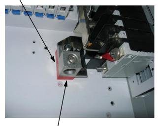
Reinstall PV Positive Output box lug in its original position using a 7/16" boxwrench. See torque chart on page 4. Install sealed 10-32 X 3/8 screw through bottom into red insulator brass insert
