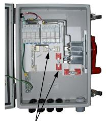
Remove Positive and Negative blocks and set aside. This is to provide access for the next steps. Step 2: Remove Positive Output busbar
