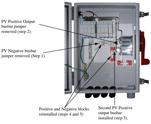
When you have finished the conversion it would be a good idea to compare your result with the photo (Left) to be sure that all steps were completed correctly. You should now have two separate four string combiners in one box. This example has one MNSPD. Refer to the wiring diagrams beginning on page 17 For adding a second MNSPD (sold separately).
