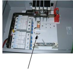
Install busbar on switch as shown.
