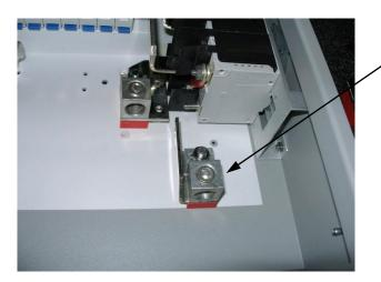
Install PV Positive Output box lug on bottom position of switch. See torque chart on page 4. Finally, replace the PV Negative busbar removed in step 1 and install busbar.
