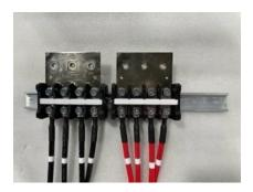
Connect the included battery-to-combiner power cables to the busbar, if not pre-wired. Use red for positive and black for negative, taking care not to reverse these cables. If the battery-to-busbar power cables are pre-wired, remove any cables which will not be used. Only install the correct number of battery cables, equal to the number of eFlex batteries. Torque the connections to 7-9 ft lbs / 10-12 Nm.
