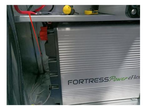
Cable connecting the invertor and busbar (2/0AWG): max bend
