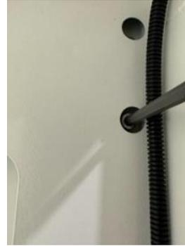
Set the upper inverter cabinet on top of the lower cabinet and then affix the two cabinets together using provided 8 attachment screws. **Do not perform this step with the batteries or inverters inside the cabinet.**
