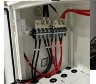
The combiner block provides 3 positions for connecting 2/0 using 5/16 lugs. The combiner block also provide 2 positions for low current connections supporting Flex Tower Fan and Guardian Power. You may double lug on either of these lower power connections, or single lug. **MAKE ALL OF THESE CONNECTIONS TO THE COMBINER BEFORE INSTALLING EFLEX INTO THE LOWER BATTERY CABINET.**
