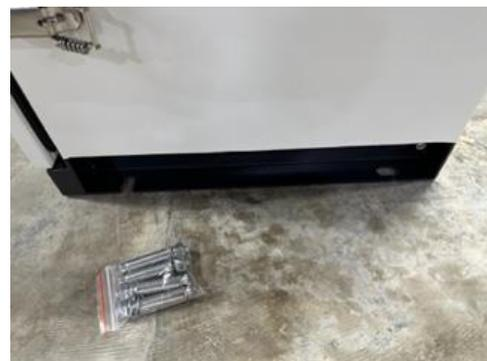
The DuraRack cabinet contains a floor plate that allows for ground mounting using M10 bolts.
