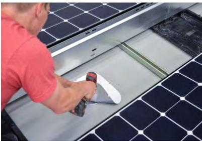
4. Slide Strut away and install Roof Attachment per manufacturer's instructions.
