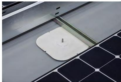
5. Slide Strut back into position over Roof Attachment.
