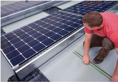
1. Position Strut under and near center of PV module in line with center slots on Wind Deflector. Position Strut throughout the array as shown on array design layout.
