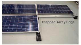
**Example of one configuration of Stepped Array.** At array edge, South Row has one less PV module than North Row, creating s stepped edge. Alternatively, Stepped Arrays may have the single PV module on the North Row.
