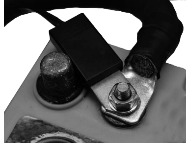
Fig 2.5(b) Temperature Sensor Installation
