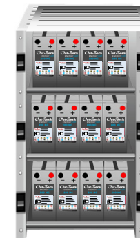
EnergyCell 200NC batteries
