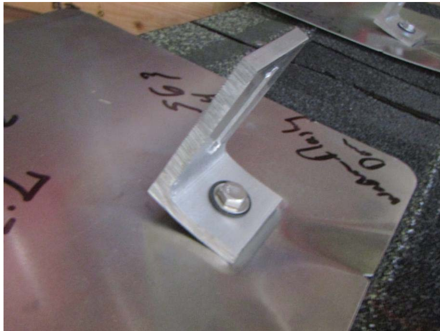
Photo 10: Lateral Parallel to Rafter Eccentric Load (post-test) - Upslope
