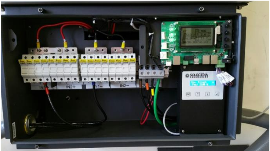
Figure 8.3 – SolrenView Monitoring Installed Inside Wiring Box
