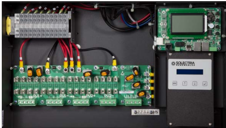
Figure 14.1 – SolrenView Monitoring Installed Inside Wiring Box
