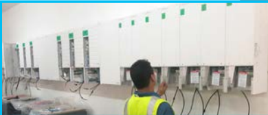
Puerto Rico Microgrids 100 schools are powered by Microgrids through Red Cross's community resiliency project Solution: microgrids using XW+ inverter / chargers, MPPT 60/80 charge controllers and other communication devices.
