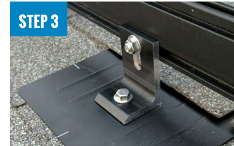
ATTACH L-FOOT TO RAIL
