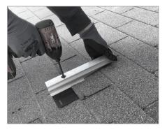
**INSTALL FASTENER & TIGHTEN:** Install fastener with sealing washer. Swivel the slider to gauge proper torque when driving the fastener. Tighten until slider stops swiveling easily.
