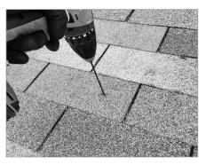
**DRILL PILOT HOLES:** Holding the drill square to the rafter, drill 3" deep pilot hole into center of rafter using 1/8" aircraft extension bit for 5/16" GRK or Unirac Custom Structural Screw, or 7/32" aircraft extension bit for 5/16" lag.
