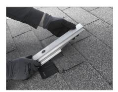
**PLACE SLIDER:** Place slider with assembly over the flashing flute, ensuring that the slider sits flat on the flashing surface.
