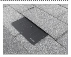
**POSITION FLASHING:** Slide the flashing up underneath the 2nd course of shingles, so that the bottom edge of the flashing does not overhang the downslope edge of the 1st course of shingles.
