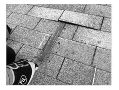
**PREPARING SHINGLES:** Use roofing bar to break seals between 1st and 2nd, and 2nd and 3rd shingle courses. Be sure to remove all nails to allow correct placement of flashing. See SFM installation guide for proper flashing placement.
