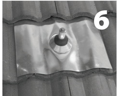
Install the 18"x 18" flashing. Pre-bend the flashing to follow the contour of the tile if curved. Apply sealant where post and flashing meet, and install EPDM counter flashing collar. Seal off the post from weather exposure with the racking hardware in the interim before racks are installed.
