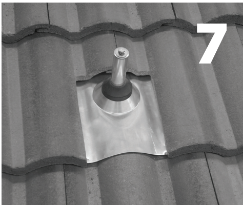
Another acceptable method is to notch the tile and install the 18"x18" flashing under the tiles. This is very common in standard roofing.
