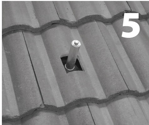
With a diamond blade on a grinder or skill-saw, cut tile to allow post to pass through. Place cut tile back in position. Insert post and tighten into place.
