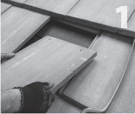
Remove tile at selected location of mount.
