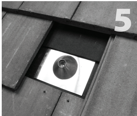
Carefully clean the building paper then install sub-flashing. Waterproof at underlayment level according to roofing manufacturer instructions and TRI Roofing Institute Guidelines.
