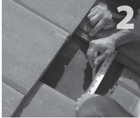
Locate and mark center of rafter.
