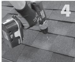
Using drill with 7/32" bit, drill pilot hole into roof and rafter, taking care to drill square to the roof. Do not use mount as a drill guide. Drill should be 'long style bit', aka 'aircraft extension bit' to drill a 1¾" deep hole into rafter.
