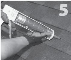
Clean off any sawdust, and fill hole with sealant compatible with roofing materials and EPDM rubber.
