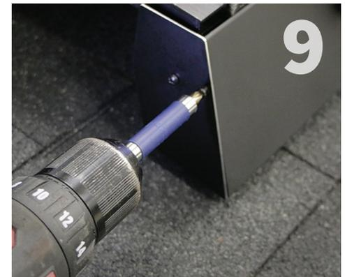
Attach End Caps with the provided screws, screwing through the holes on the end cap with a #2 Phillips screwdriver, into the screw bosses of the extrusion insuring the black side of the Skirt End Caps is facing outward.
