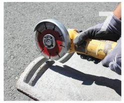
Cut a clearance notch in the weather guard lug using a grinder with a tuck point blade. Make sure the tile seats back down in it's original position. Leave at least ¼" of tile to prevent breaking through.
