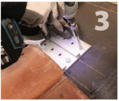
Connect hook to base plate and drive lag screws into rafter through the two holes to a solid, snug fit. DO NOT over tighten lag screws, this may compromise their holding strength.
