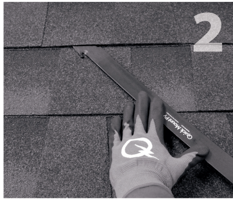
2 Lift composition roof shingle with roofing bar, just above placement of conduit mount.
