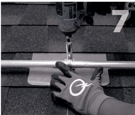
7 Insert lag through hole in block, and position clamp over conduit. Using drill with 7/16" socket, drive lag until block is tight.
