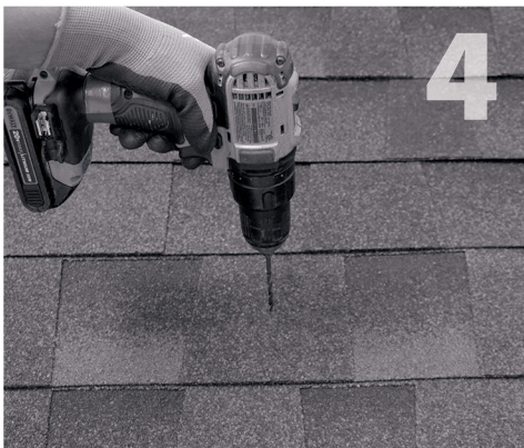
4 Using drill with 1/8" bit, drill pilot hole into roof taking care to drill square to the roof. Do not use mount as a drill guide.
