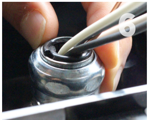
Install Grommet: Slide the grommet over the wires and push it down into the conduit such that it extends over the cut edge and locks into itself. The grommet should extend over the top and be secured to the conduit. It should not be loose.
