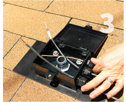
Install PV Wires: Pull PV system wiring through the cord grips and tighten the cord grips to seal around the wires making a watertight connection. Ensure each wire has a minimum of 6" of lead inside the box per NEC requirements.
