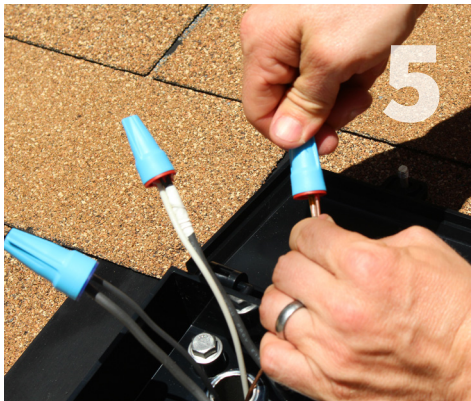
Connect Wires: Install the supplied wire nuts to achieve one of the approved wiring combinations outlined in Section VI.
