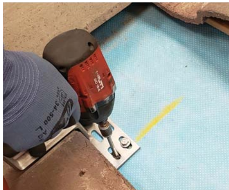
5. Reposition hook, secure with included lag screws.
