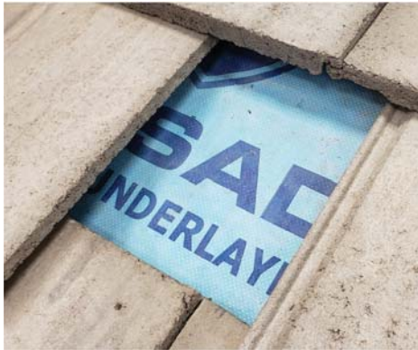
1. Remove tiles around installation area.
