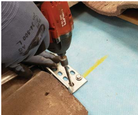
5. Reposition hook, secure with included lag screws.
