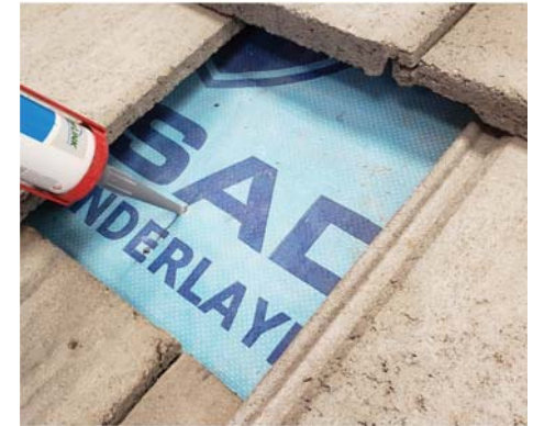
4. Remove hook, clean debris, then fill pilot holes and rib on back of hook with roofing sealant.
