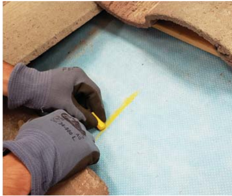
2. Locate and mark rafters.
