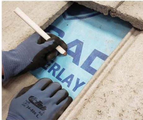
2. Locate and mark rafters.
