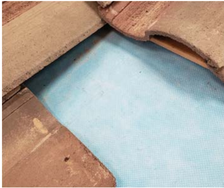
1. Remove tiles around installation area.
