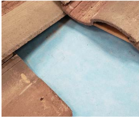
1. Remove tiles around installation area.
