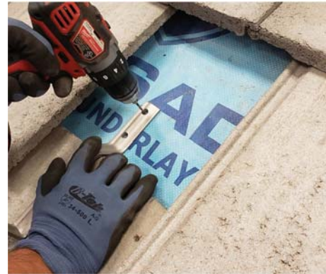
3. Position hook. Use 3/16" bit to drill 2 pilot holes.
