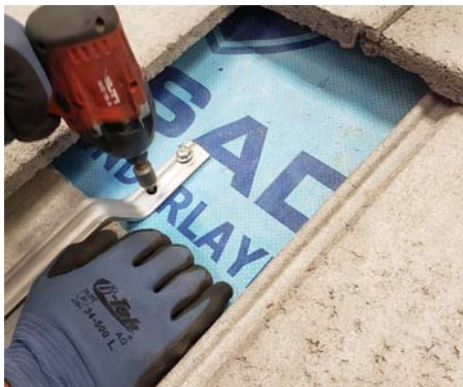
5. Reposition hook, secure with included lag screws.
