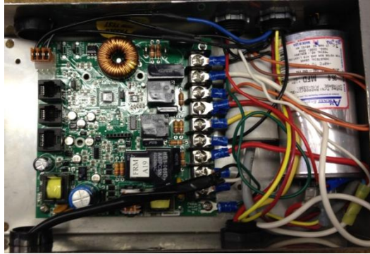
FX II completed installation
