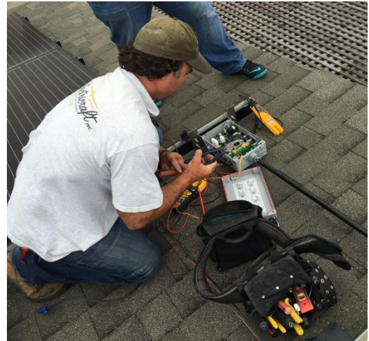
Figure 1: Fronius Rapid Shutdown Box installation
