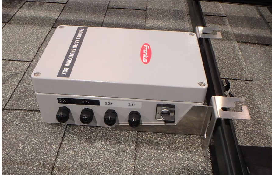
Figure 5: the bracket is in contact with the rail top, but the RSB is touching the roof. Therefore, the RSB needs to be raised by either adjustable attachment to the side rail or by raising the rail itself.
