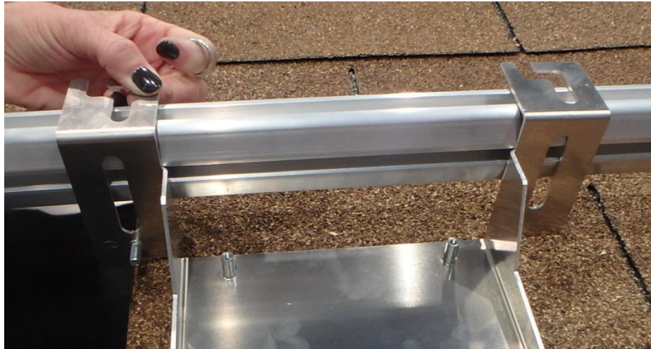
Figure 3: A generic rail system demonstrates typical top and side channels for mounting bolts
