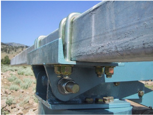
TIGHTEN NYLOCK 5/16" U-BOLT NUTS EVENLY .
