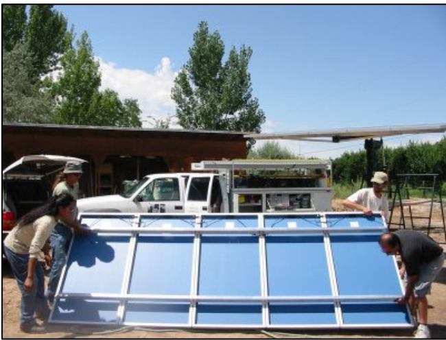
Sub-Array Approach: Requires a lot of people power. Notice that the rails bolt to the intermediate module holes. Lift by the tracker rails only, not the module frames!
