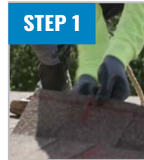
LOOSEN SHINGLES
