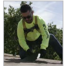
PLACE FLASHING
