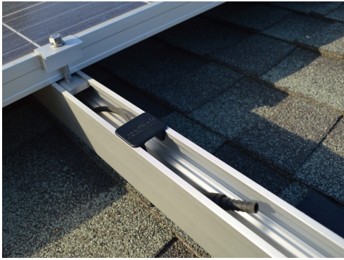
Wire Clip Installed
