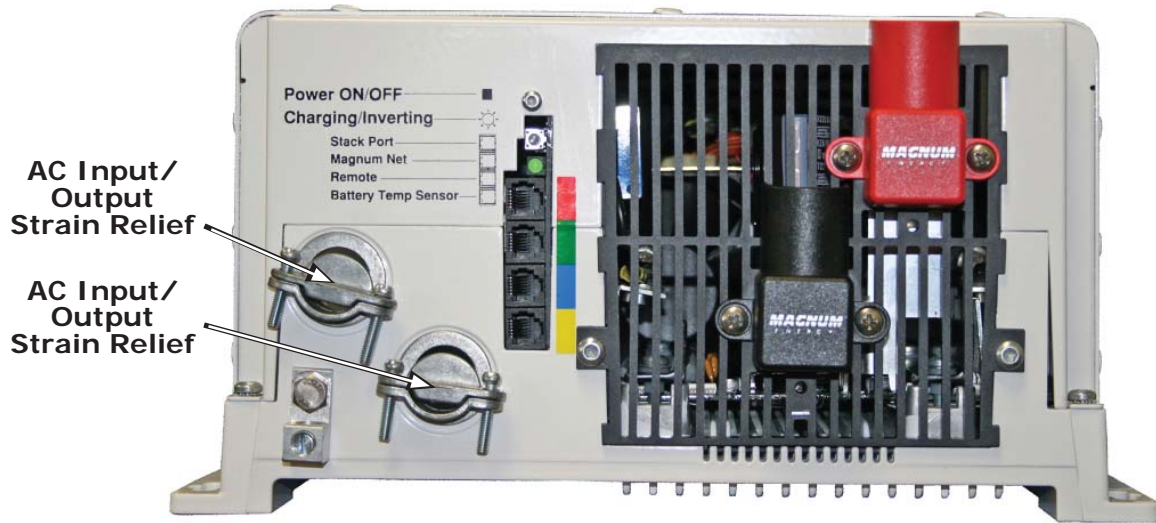
Figure 2-8, MS-E Series Inverter/Charger - AC Wiring
