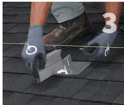
To adjust in 1/4" increments move the top slider up or down one notch. To adjust in 1/8" increments rotate the top slider 180 degrees. Repeat for the other mounts until top slider elevations are uniform across the row.
