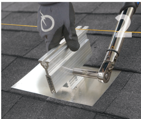
The string acts as a guide for aligning the top slider positions of all the mounts in the row. To adjust top slider height, remove machine bolt, separate top slider from QBlock slider and reinsert at proper location. Use torque wrench 1/2" socket to torque all top slider bolts to 6 ft-lbs.
