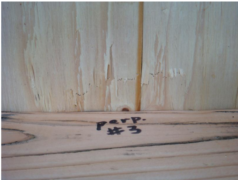
Figure 4. Buckled Plywood Shear Perpendicular to Rafter
